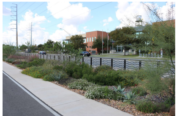
Low Impact Design (LID) bioswale in parking lot at 1902 S. Alamo.
